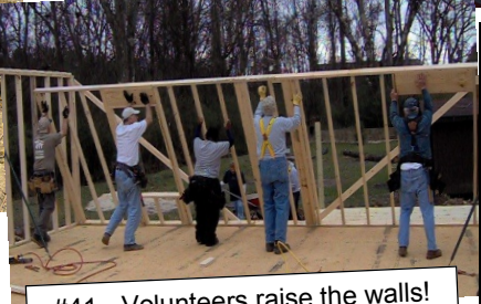
#41 - Volunteers raise the walls!
